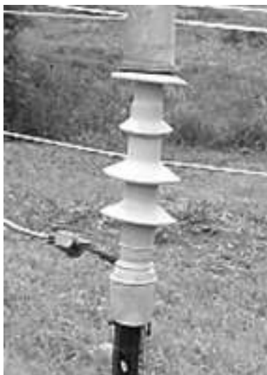
FIGURE 13.6 Cold shrink termination with skirts.
