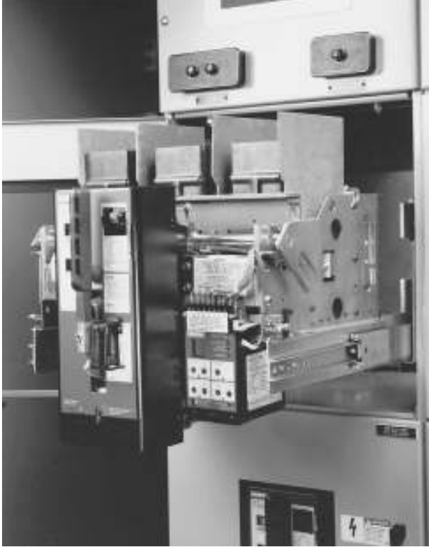
FIGURE 3.11 Low-voltage power circuit breaker racked completely away from the bus. (Type RL circuit breaker manufactured by Electrical Apparatus Division of Siemens Energy and Automation, Inc.)
