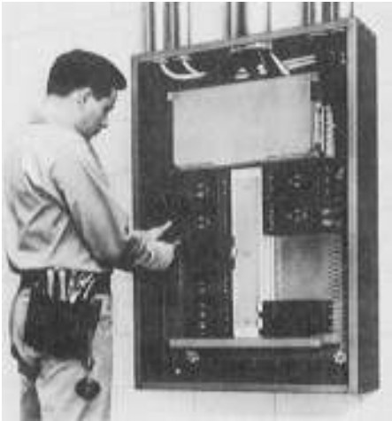
FIGURE 3.13 Panelboards equipped with molded-case circuit breakers. (Courtesy McGraw-Hill, Inc.)
