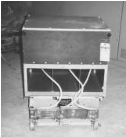
FIGURE 2.67 Front view of a 15-kV grounding switch. (Courtesy UNO-VEN Refinery, Lemont, IL.)
