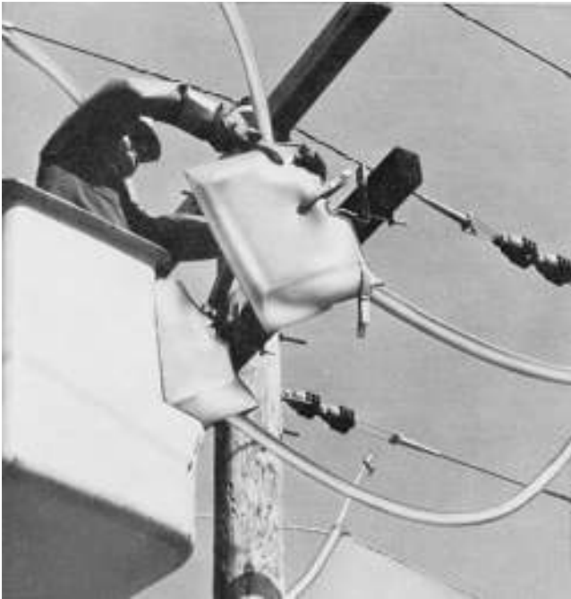
FIGURE 2.17 Typical insulating rubber covers. (Courtesy W.H. Salisbury and Co.)
