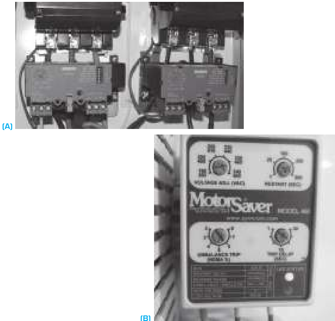
FIGURE 13–10 (A) Electronic overloads for motor controllers. (B) Voltage monitor to save motor from damage caused by voltage variations.
