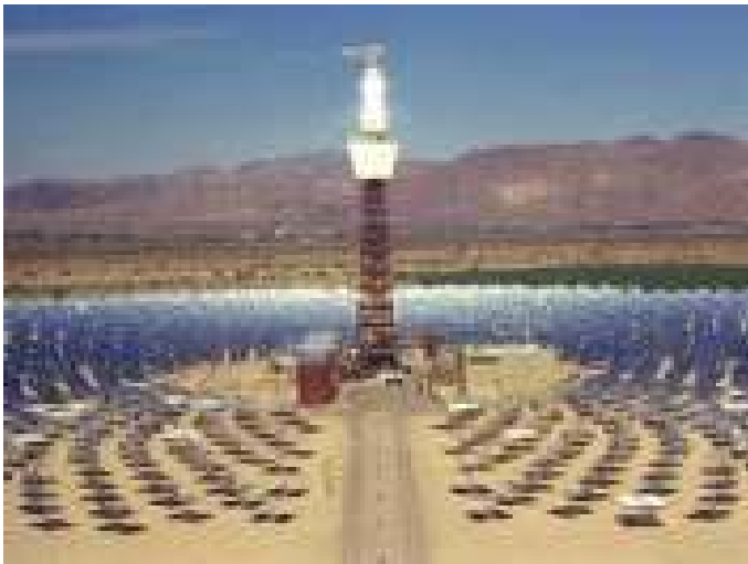
FIGURE 3.7 A solar thermal installation. Source: http://www.photovoltaicsolarenergy.com .
