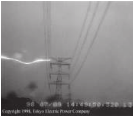
Figure 21.1 1000 kv design Double-Circuit Transmission Line (TEPCO, Kita-tochigi line, 427km)
