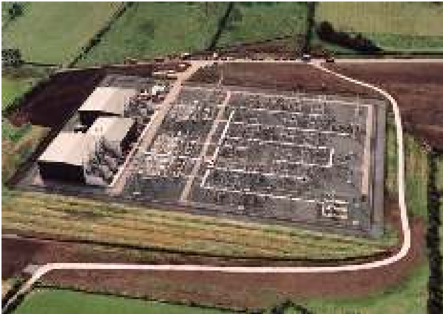
Figure 1.2 Terminal station of Moyle HVDC interconnector (Bipole 2 \times 250 MW, \pm 250 kV, with light triggered thyristors, commissioned in 2001). Reproduced with permission of Siemens.
