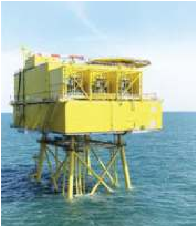
Figure 21.6 Offshore platform for BorWin1 HVDC (2012). Reproduced with permission of ABB.
