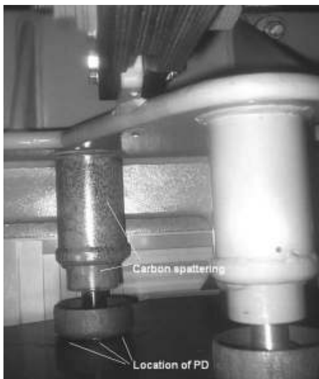
Figure 21.24 Transformer internal partial discharge from a core clamp
