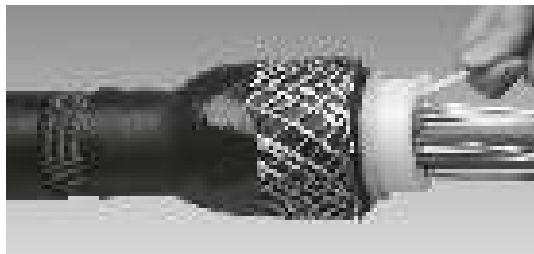
Figure 7.1.1-7: Assembly of a permanent elastic joint by cold-shrinking technique: Joint (including outer tube) that is pre-stretched and present on a spiral is arranged over the connecting point and is lowered by pulling out the spiral (left to right in the image), Figure 7.1.1-6 shows a section after the assembly. Photo Tyco Electronics, now TE Connectivity.
