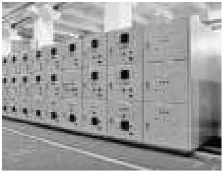
FIGURE 7.1 Medium-voltage switchgear
