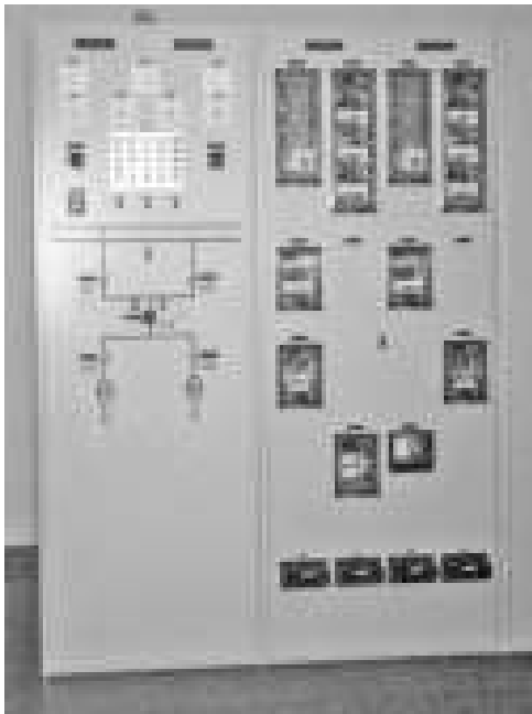
FIGURE 12.13 Steel panel with electromechanical relays and control panel
