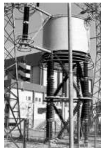
FIGURE 30.8 Installation of an air-cooled smoothing reactor.
