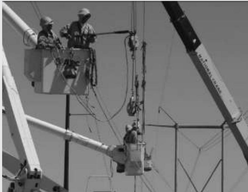
Figure 4 Re-conductoring a 345-kV line.
