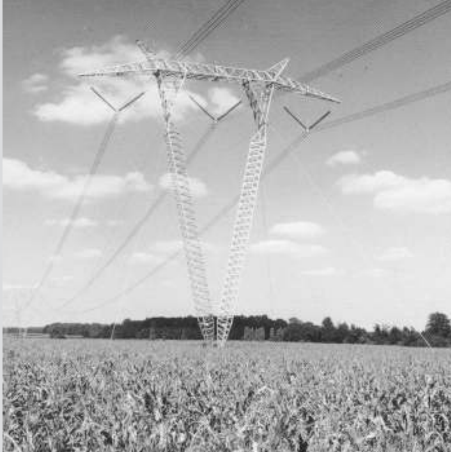
765-kV transmission line with aluminum guyed-V towers (Courtesy of American Electric Power Company.)
