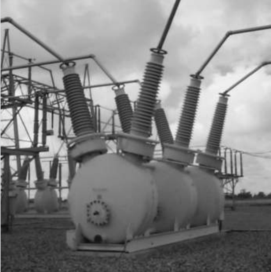
345-kV SF6 circuit breaker installation at Goshen Substation, Idaho Falls, Idaho, USA. This circuit breaker has a continuous current rating of 2000A and an interrupting current rating of 40 kA (Courtesy of PacifiCorp.)
