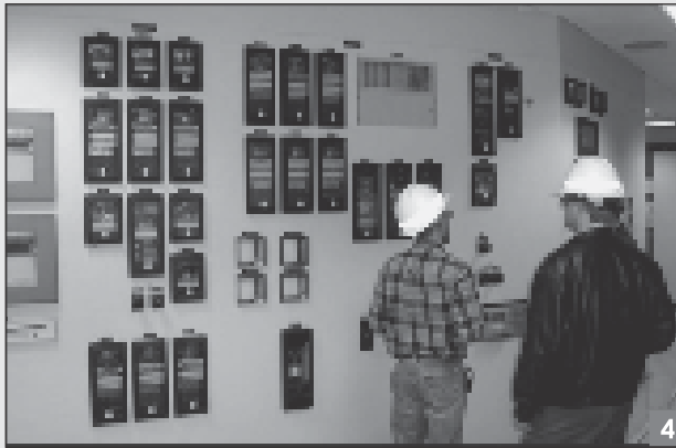
Figure 4 The old EM transformer differential relays (Photo courtesy of Basler Electric Company.)
