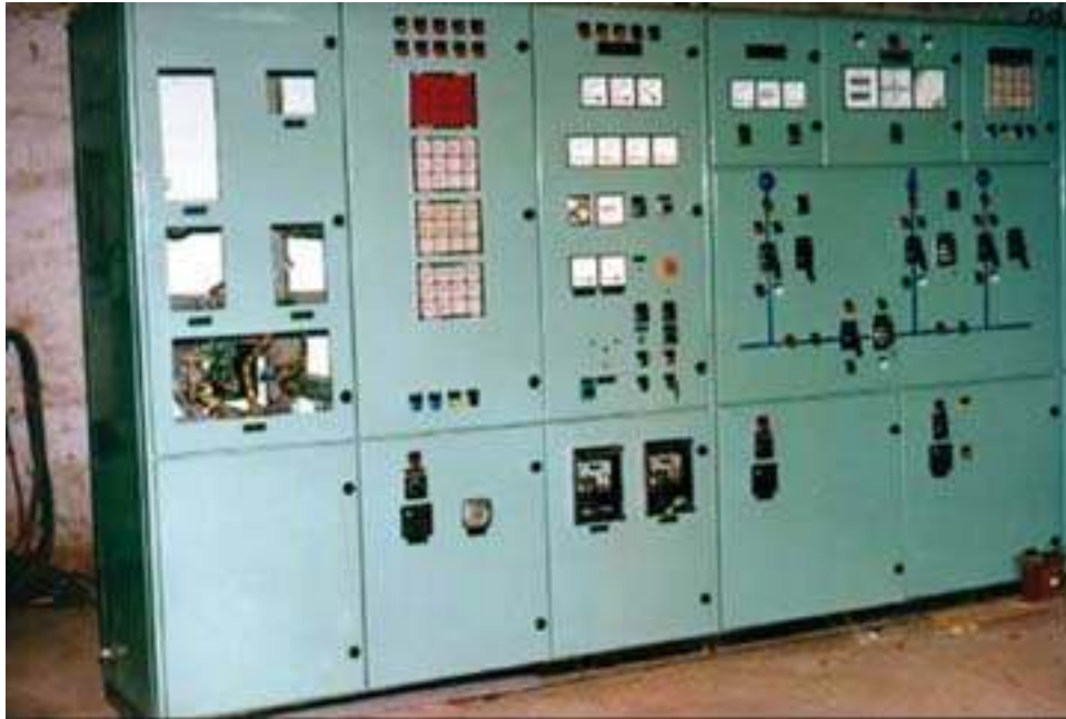
Power Factor Improvement
