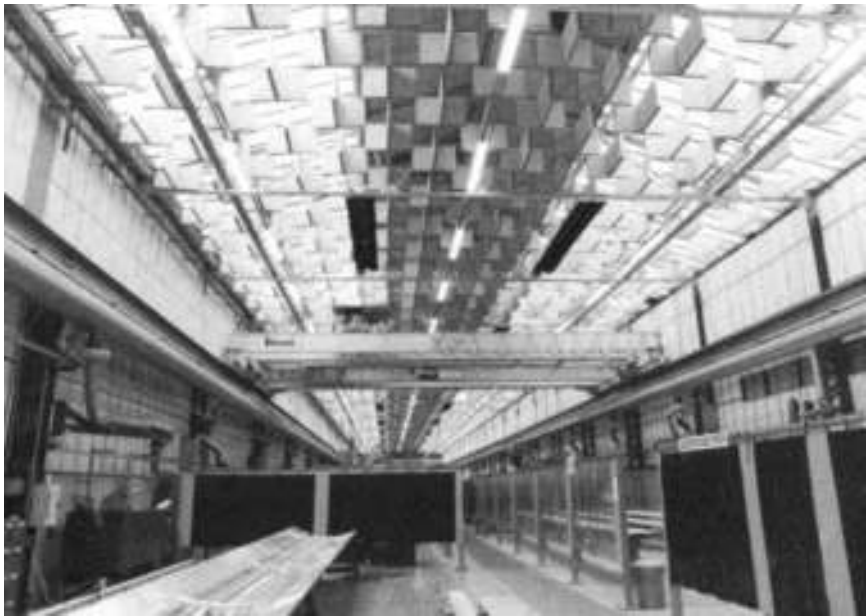
Figure 3.5.14 Acoustic absorption treatment showing suspended panels and wall treatment (Courtesy Ecomax Acoustics Ltd)
