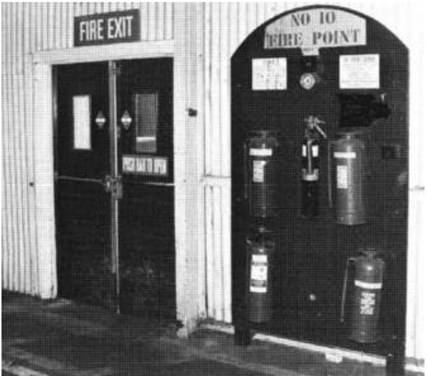
Figure 4.2.5 Clear unobstructed fire point (Courtesy Reed Medway Sacks Ltd)
