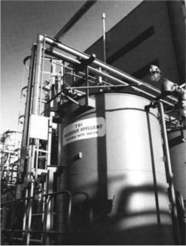
Figure 4.7.3 Storage tank for non-flammable liquids (Courtesy Rhône-Poulenc-Rorer)
