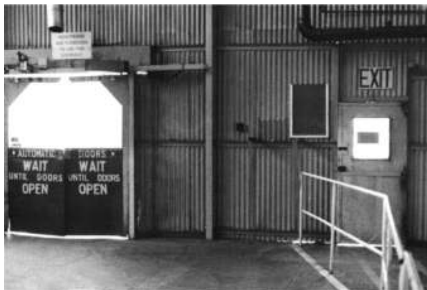
Figure 4.3.17 Separation of truck and pedestrian gangways
