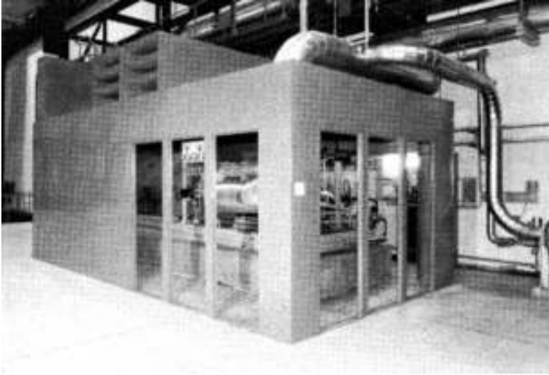
Figure 3.5.10 Noise enclosure. (Above) cross-section through typical noise enclosure wall; (below) noise enclosure with access doors removed (Courtesy Ecomax Acoustics Ltd)
