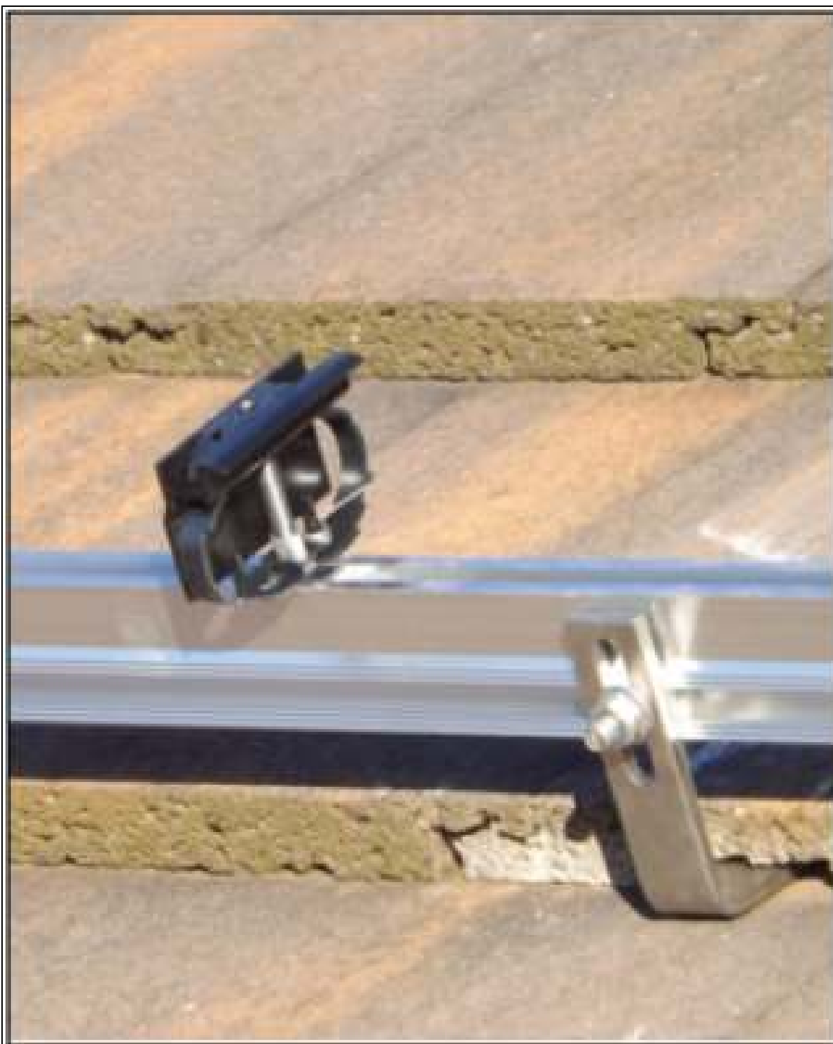
Above: Close up of a roof-mounted system, showing a roof hook, the mounting rail and a solar panel clamp.
