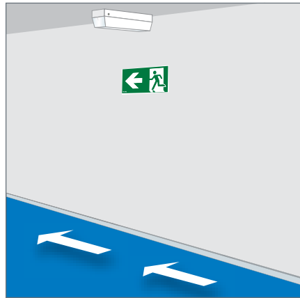
All safety exit signs
