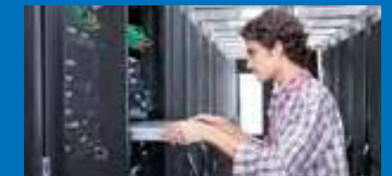
Backup Power UPS
