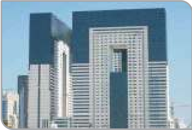
Dafna Tower 3&4, Doha
