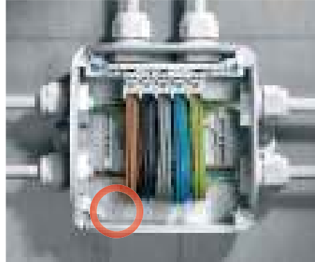
Open condensation water membrane
