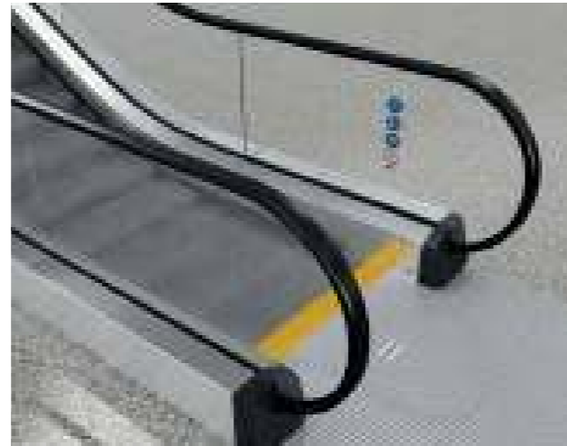
Figure 5.15 A glass balustrade is an attractive option for shops and airports
