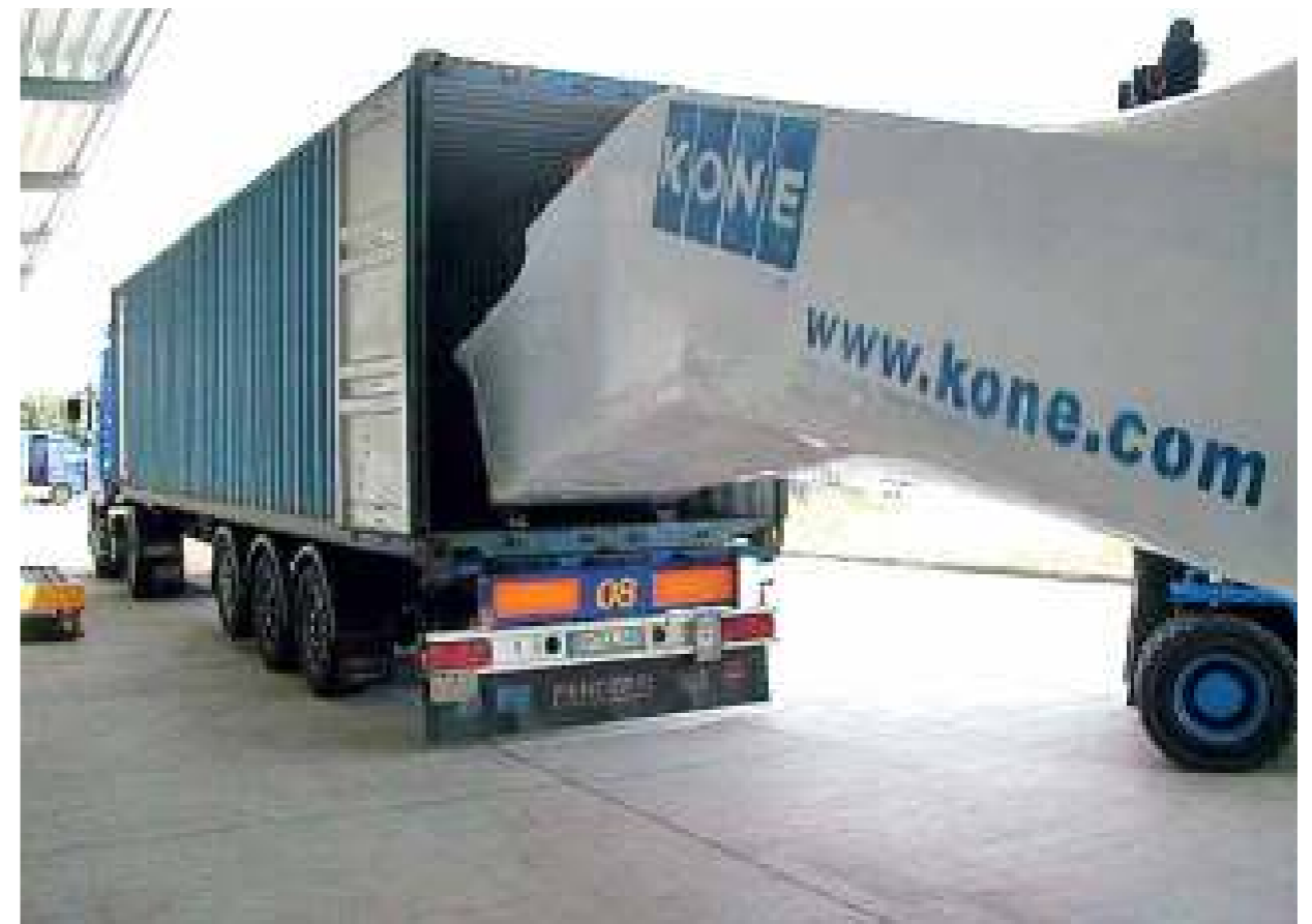
Figure 7.7 Unloading an escalator using forklift trucks
