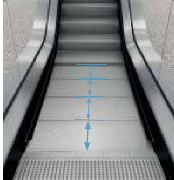
Figure 5.10 Horizontal steps enable a passenger to step safely on and off the escalator.
