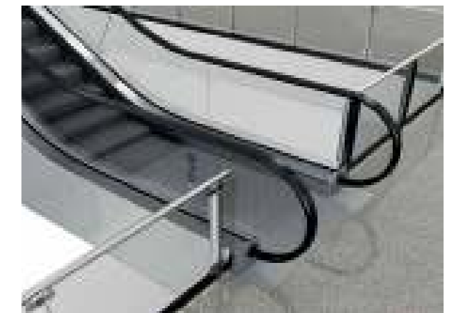
Figure 5.19 An extended balustrade allows railings to neatly butt against the escalator balustrade
