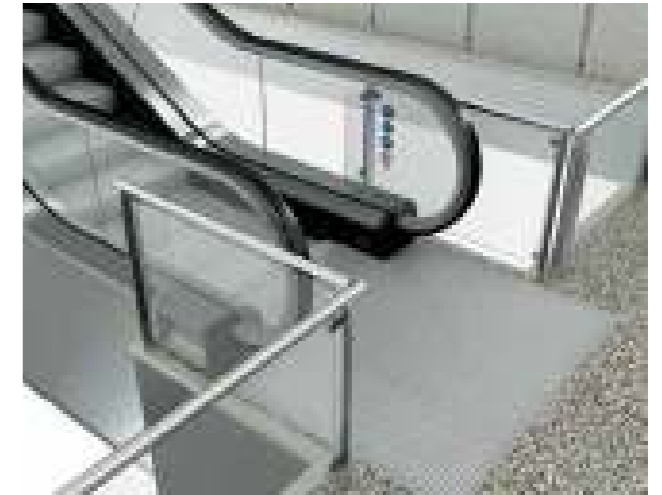
Figure 5.17 Standard arrangement without extended balustrade requires 90° static railings to be installed for safety reasons
