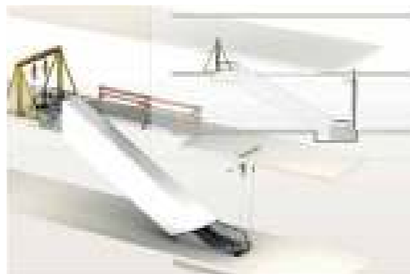
Figure 8.5 Installation using a lifting frame
