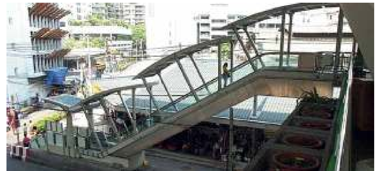
Figure 4.3 The outdoor escalator should be covered by a roof to improve passenger safety and convenience.
