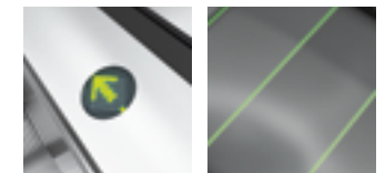
LED traffic lights located in the decking
