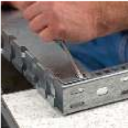
Using a screwdriver, secure assembly by bending small tab on each leg. All leg support sections can be assembled in advance or offsite for greater efficiency.
