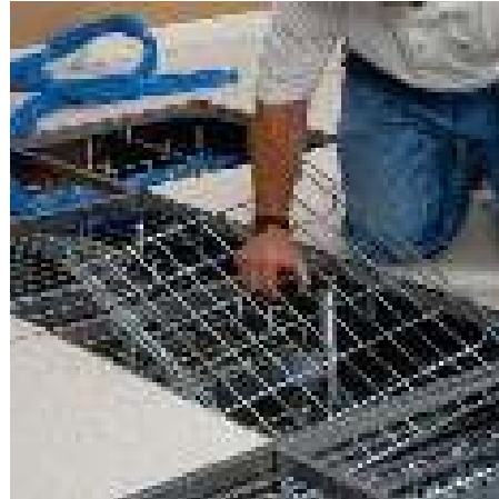
Place 2' tray sections in position.
