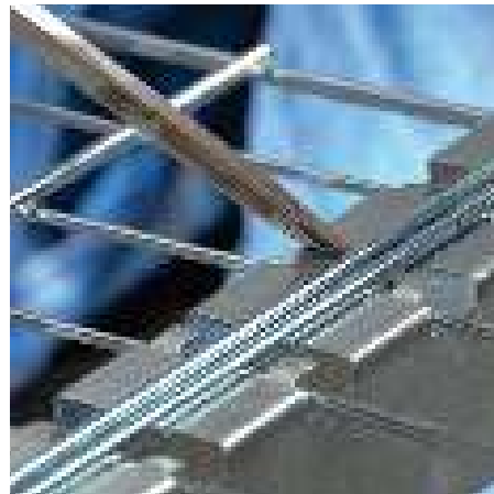
Bend FAS style tabs with screwdriver to secure tray. Double rows of FAS tabs on UFS crossbars act as tray splices.
