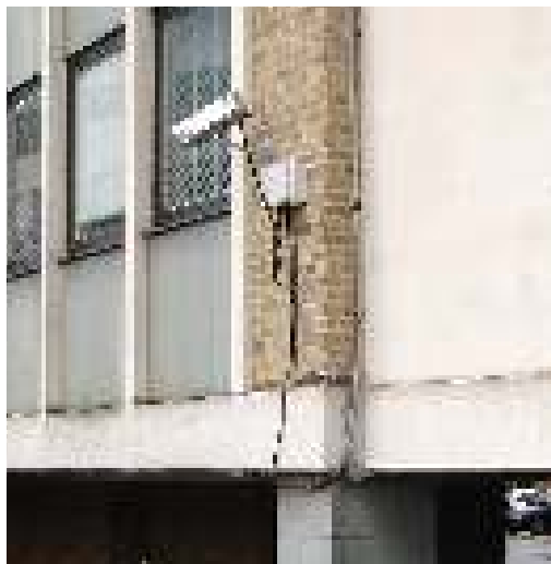
Figure 65. Conventional down-conductor separation distance problem.
