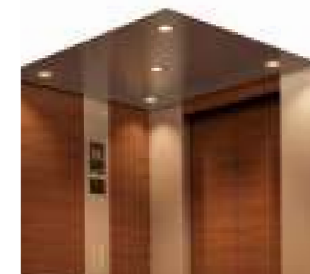
Ceiling: L210S LED downlights (yellow-orange)
