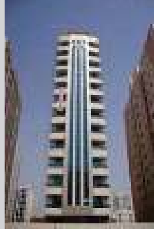
Residential Building At Al Qusaia, Dubai
