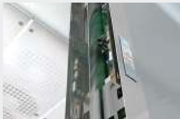
The Schindler 3100 inspection and test panel is incorporated into the doorframe at the top floor, eliminating the need for an additional control cabinet.
