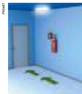
Near every fire safety device and call point.
