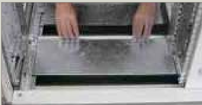
Sliding plates enable the size of the aperture to be adapted to the quantity of cables to be fed through
